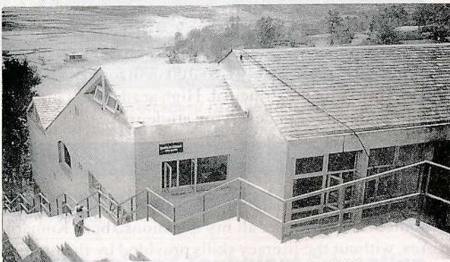
The new science building complete!
