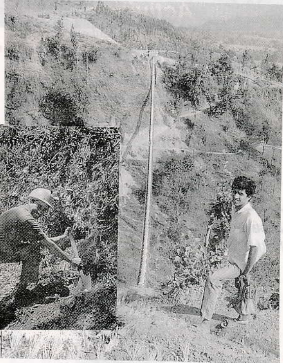
Irrigation pipeline in Andhi Khola
