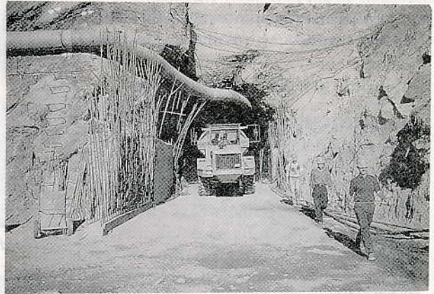
Entrance to the powerhouse access tunnel at Khimti
